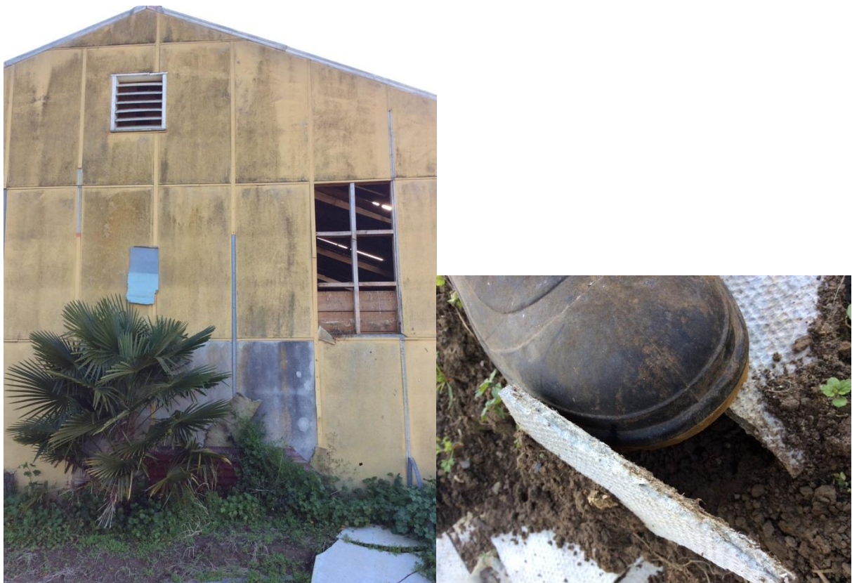
Photograph 11: Large stable/hay barn located on Property C adjacent to Mclarin Road near the entrance to Property A. AC property file information indicated that the walls may be constructed using asbestos containing material (fibre cement cladding).
